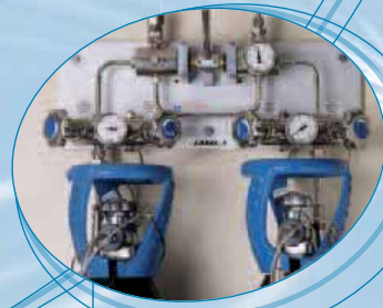
Equipment and piping installation
